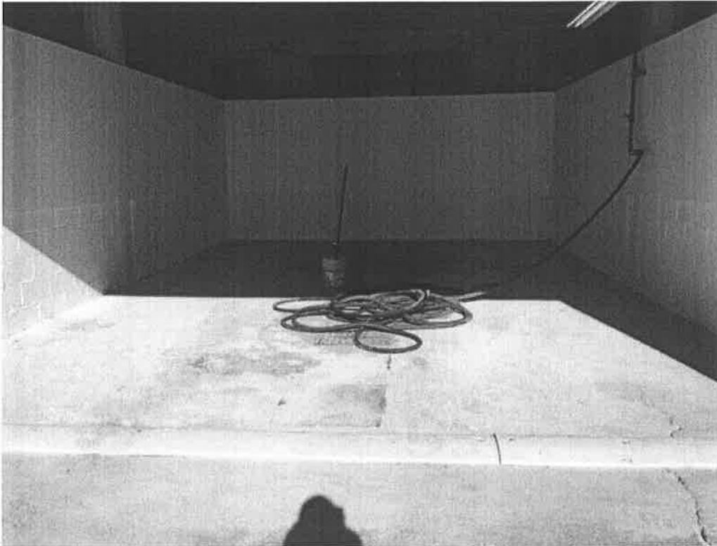
Photograph 3 – New equipment wash bay.
